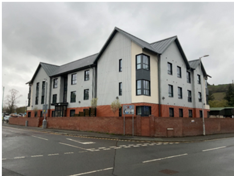
Newly built Council apartments in Newtown
